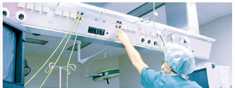
Connectors, sockets, connecting leads and multiple-pole connectors for the reliable connection of medical devices.
